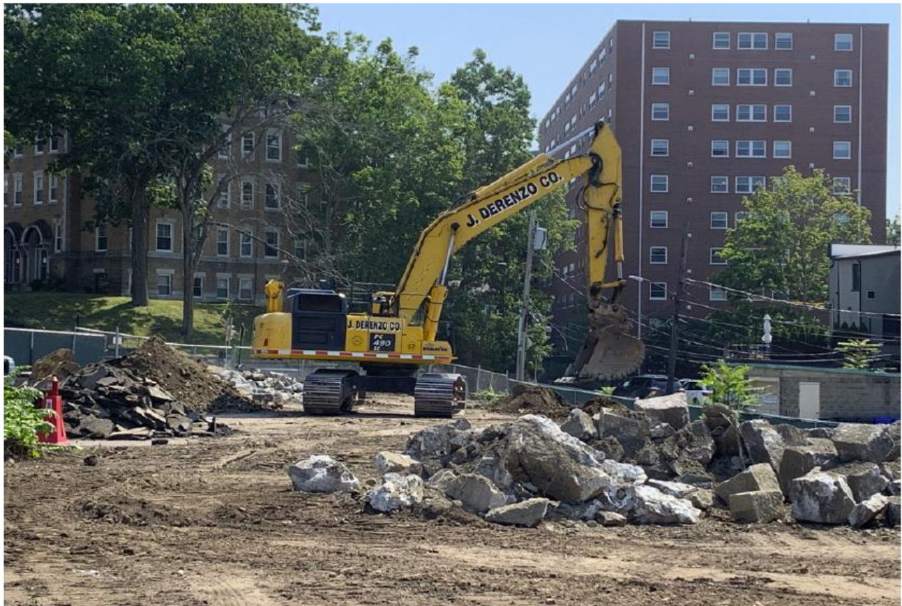
Removal of the retaining wall between the site and the alleyway
