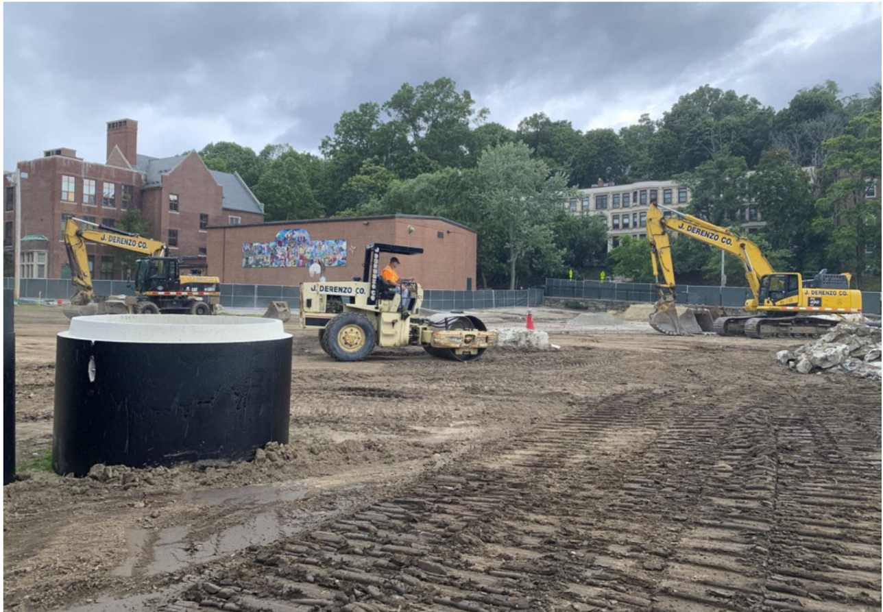
Site preparation underway
